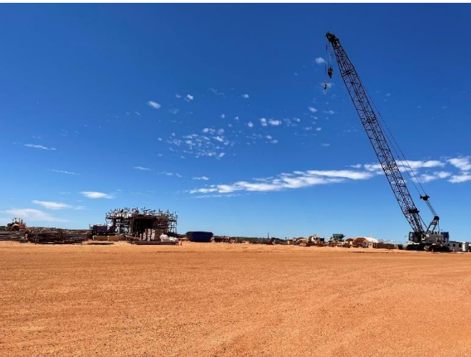
Figure 5: MSP formwork and construction
