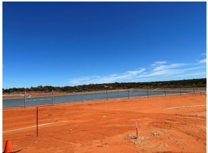
Figure 6: Water ponds filled ahead of commissioning
