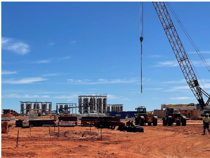
Figure 3: WCP spiral on site for installation
