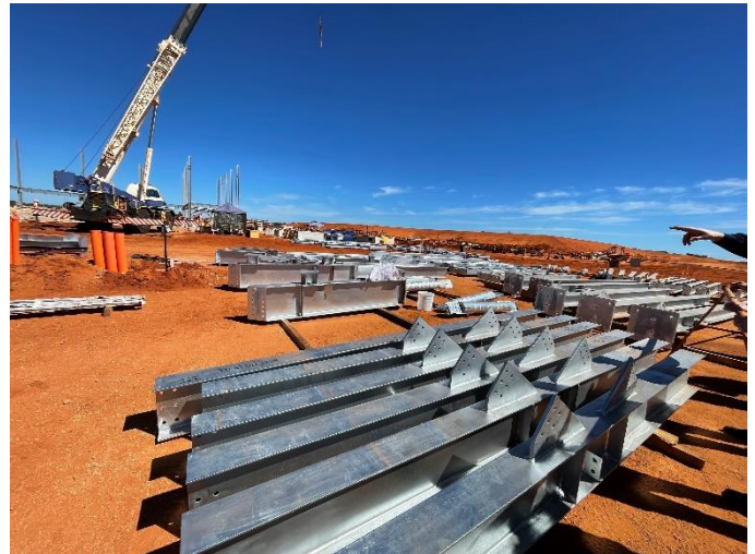
Figure 4: Structural steel ready for installation
