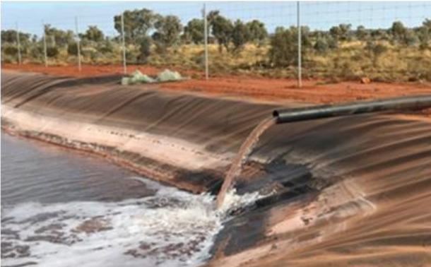
Image: Typical HDPE lined Water Pond
