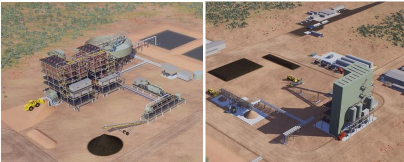
Figure 1 Coburn Preliminary 3-D Engineering Model of Wet Concentration Plant (WCP) and Mineral Separation Plant (MSP) Infrastructure
